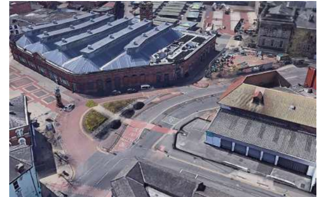
Taxi rank and compound site, Wellington Road
